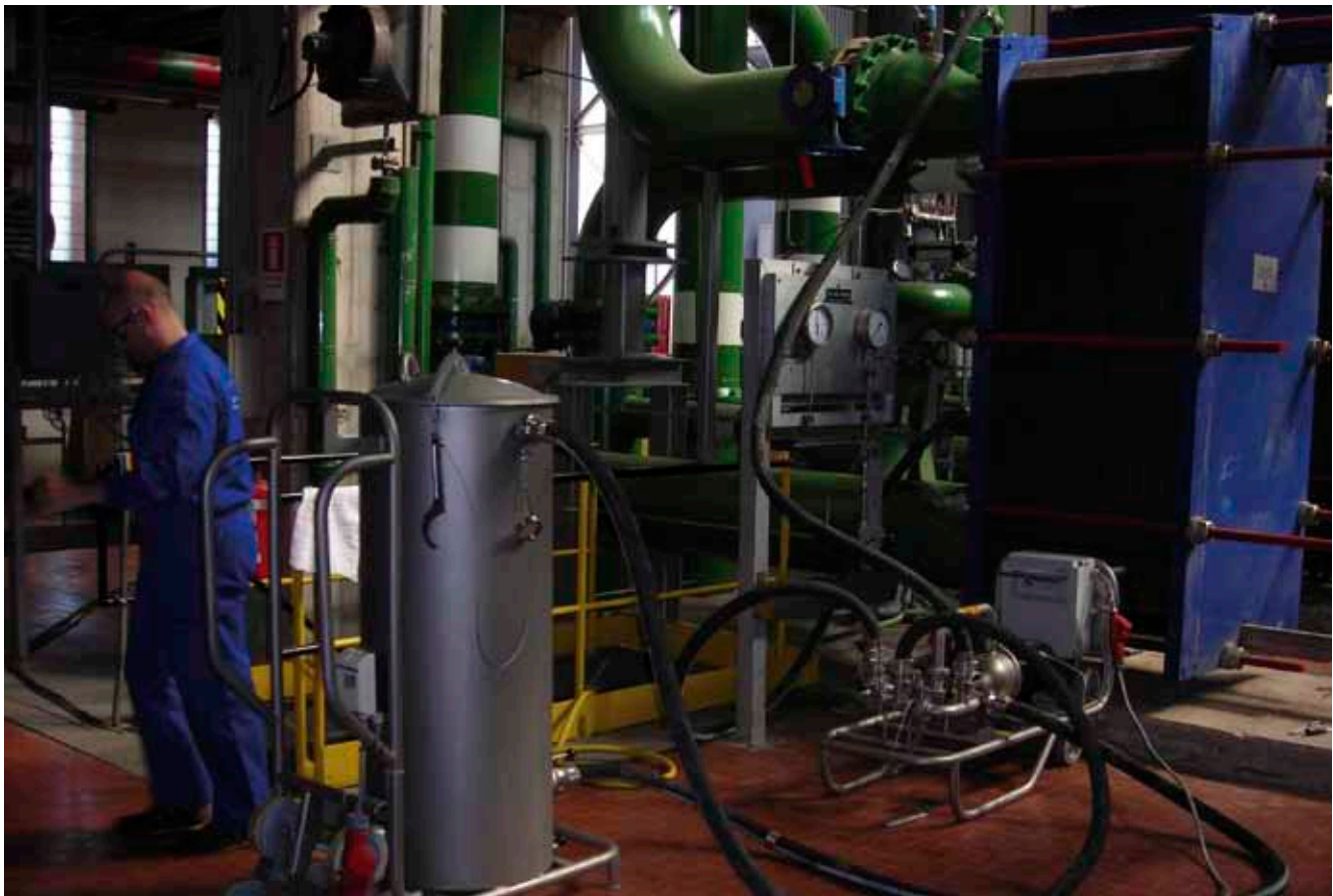
M30 heat exchanger installed at customer's plant
