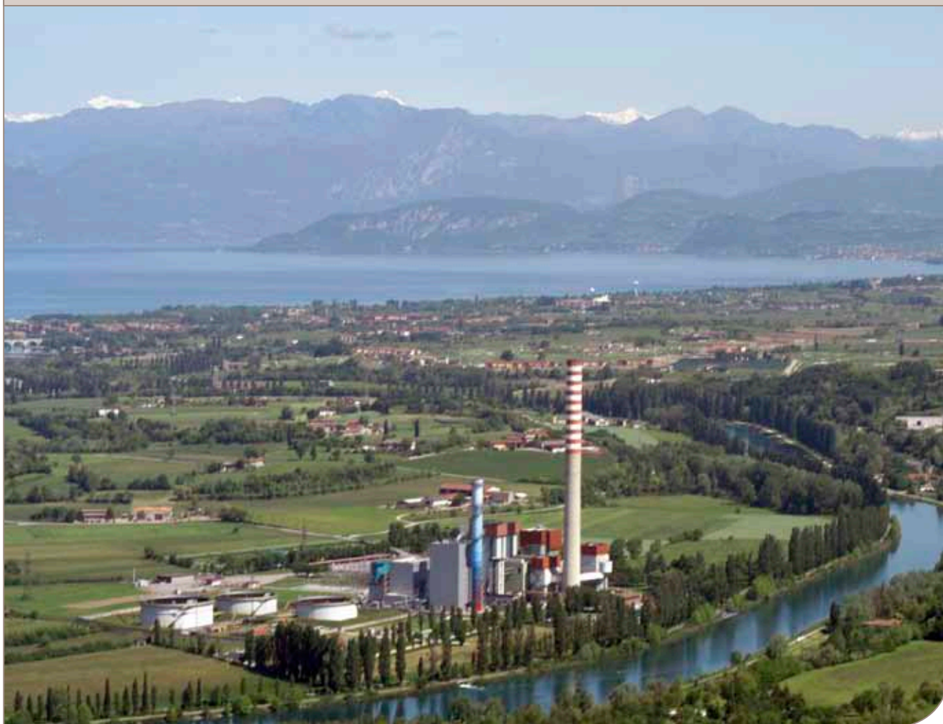
Mincio Thermoelectric Power Plant (aerial view)
