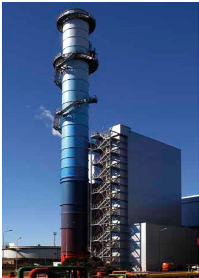
Heat recovery steam generator and chimney
