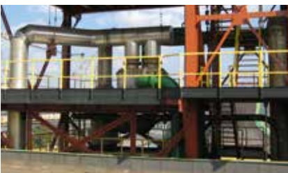
In 2003, AB Achema in Lithuania replaced its NOx gas coolers/condensers. With only 193 sqm of heat-transfer area, the Compabloc achieves the same capacity as two shell-and-tubes with a total heat-transfer area of 950 sqm.
