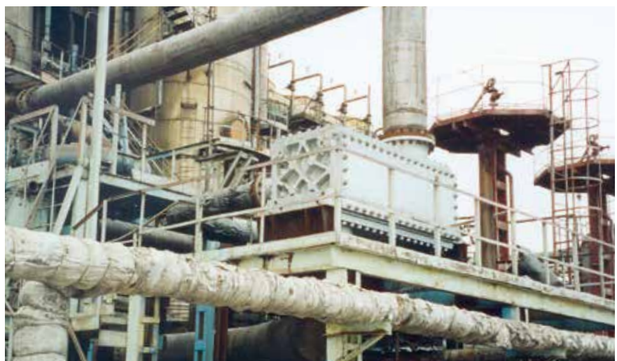
To increase production capacity, DneproAZOT, a Ukrainian fertilizer plant, replaced two shell-and-tube gas coolers with a single fully welded Alfa Laval Compabloc. The gas can now be cooled down to 35°C, even in summer, using water from the nearby Dnieper river. This has resulted in increased urea production and lower compressor power consumption.
