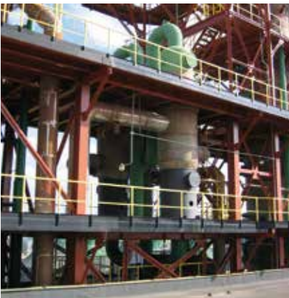
In 2003, AB Achema in Lithuania replaced its NOx gas coolers/condensers. With only 193 sqm of heat-transfer area, the Compabloc achieves the same capacity as two shell-and-tubes with a total heat-transfer area of 950 sqm.
